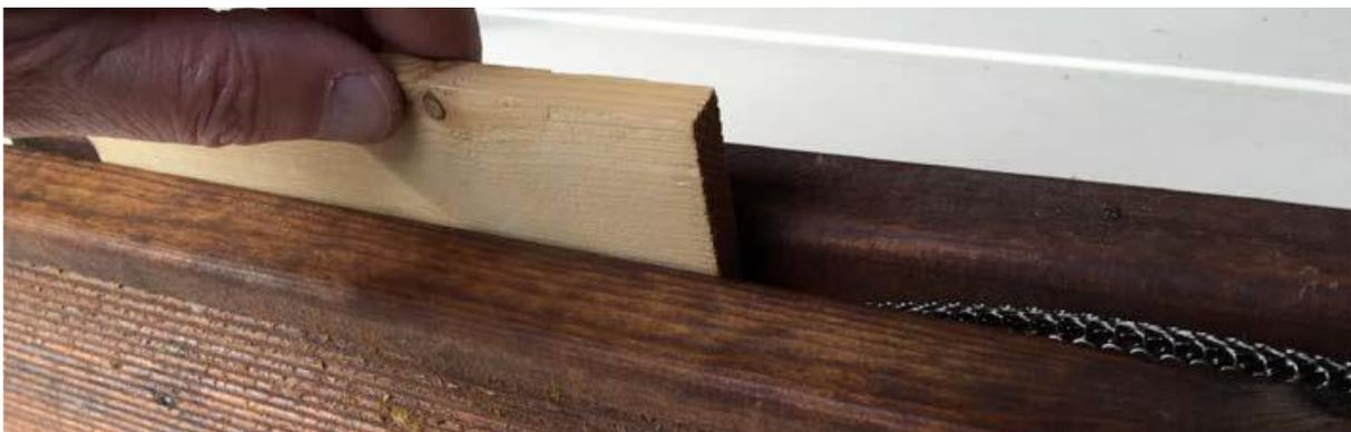
The gap vent can be used in gaps with height up to 16 mm. The gap vent is adjusted to the gap height by carefully shaping the mesh. Make sure that there are no openings between the contact surface and the vent.
